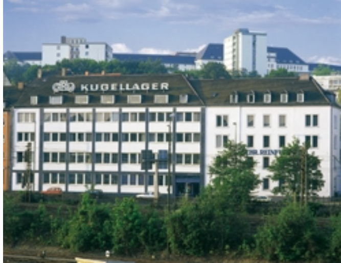
Administration and production facilities in Würzburg
